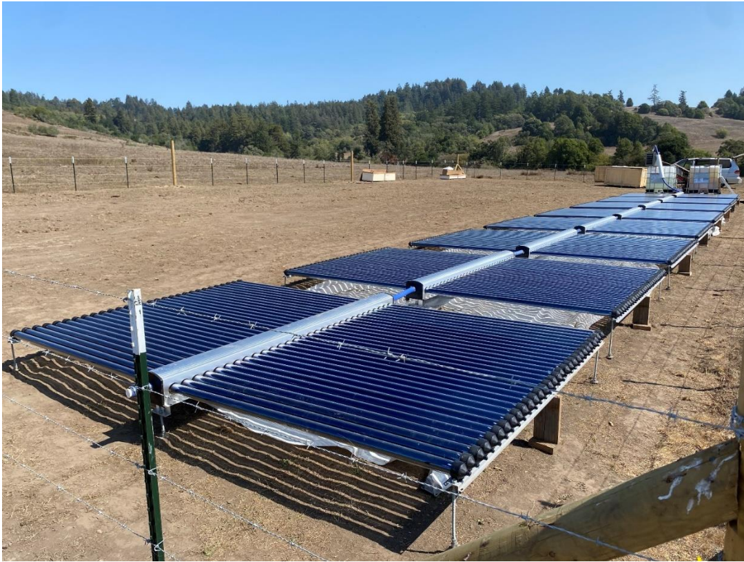
Figure 8 – Eight-Panel Steam-Generating Solar Array, Freestone, CA Installation
