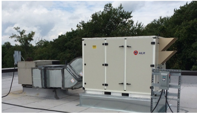
Figure 24 – The Installed LDDX-Ad Prototype
