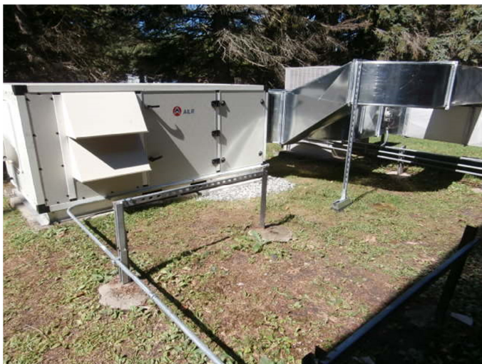
Figure 21 – The Installed LDDX-WF Prototype
